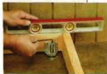
▲ Level the Base. An Allen wrench is all you need to adjust the leg levelers used on the cabinet base.
