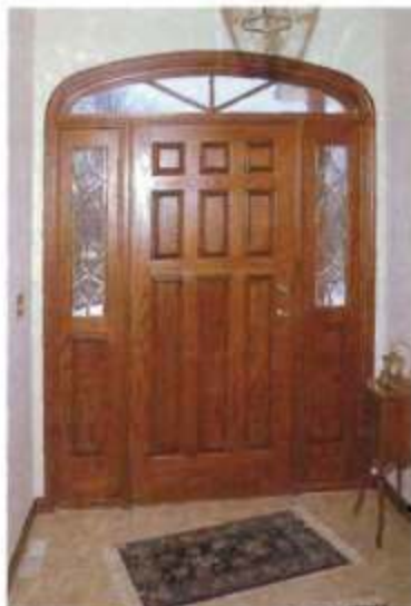
▲ A Grand Entrance. The raised-panel entry door and side lights were also made by Daryl.
