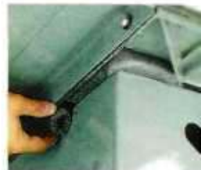
▲ To seal the upper part of the cabinet, stuff in short pieces of foam insulation between the "ribs" of the cast iron table.
