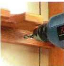
▲ The rack is held securely in place by driving screws through a cleat and into the wall.
