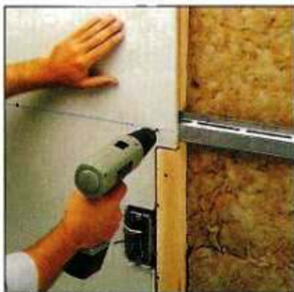
Step 4. Now you can screw a layer of drywall to the resilient channel. Use short screws so they don't hit the studs.
