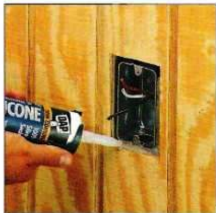
Step 6. To seal noise in, and still allow the walls to flex, fill in any gaps with a high-quality silicone caulk.
