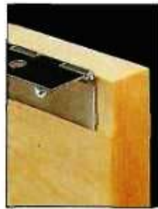
It's easy to install a piano hinge when you cut a shallow "alignment" rabbet for it to sit in.
