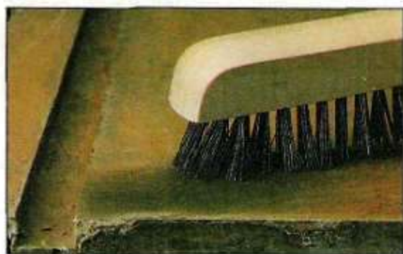
A. Remove Loose Rust. To get a better look at the condition of the top, a wire brush is used to remove most of the dirt and loose rust.
