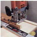
The housing is widened by inserting two pieces of the shelf board in the pockets of the Accurate Guide
