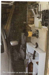
The clearance as seen from outside
