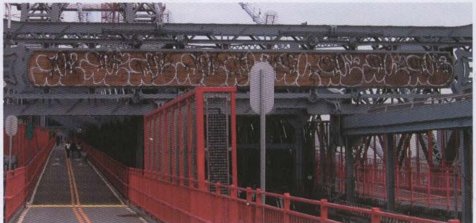
Kez 5 crossing out SI, Williamsburg Bridge April 2004
